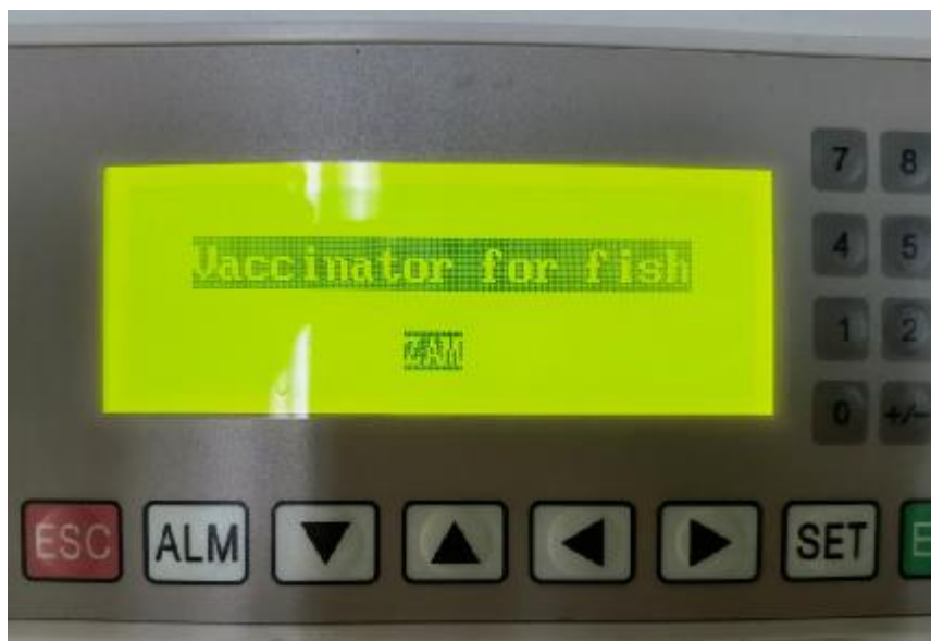
Figure 1 Interface during power-on
